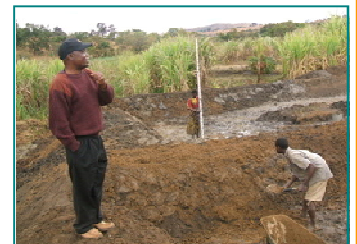
Late Mr Malukula supervising pond construction in Dowa district
